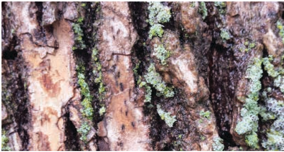
D-Shaped Exit Holes
